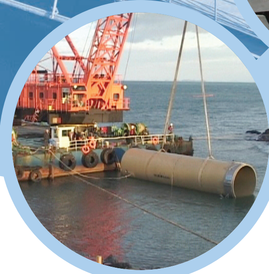
Installation of ocean bed blocks
