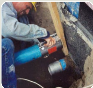
▲ U.S.: sewerage repair work
