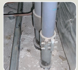
▲ PVC + Steel Pipe Connection
