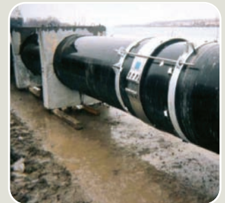
▲ U.S.: nuclear power plant
