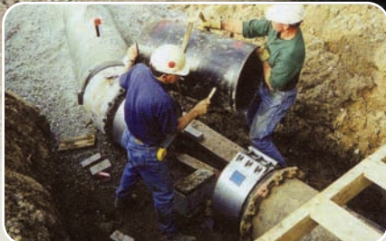
▲ Repair work for pipes replaced underground
