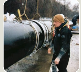
▲ UK: district heating work
