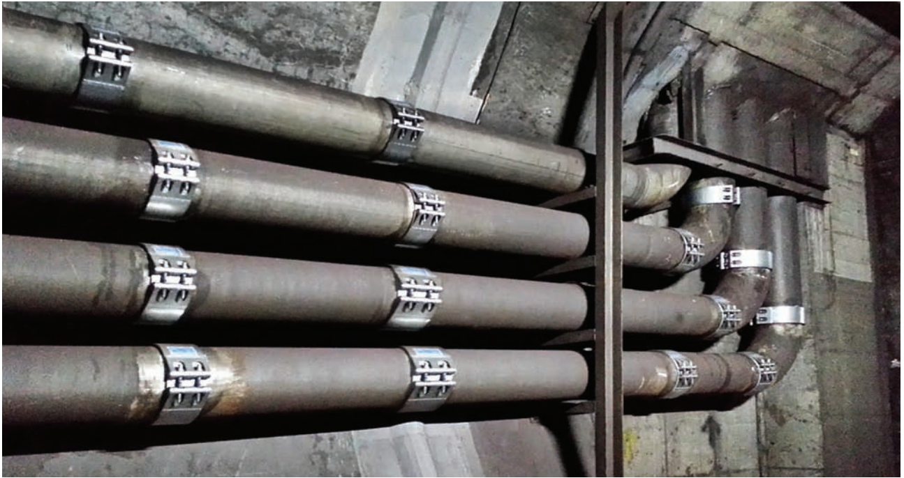
▲ Underground drainage repair(Maintenance) works
