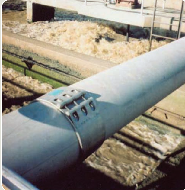
▲ Spain: water purification facilities
